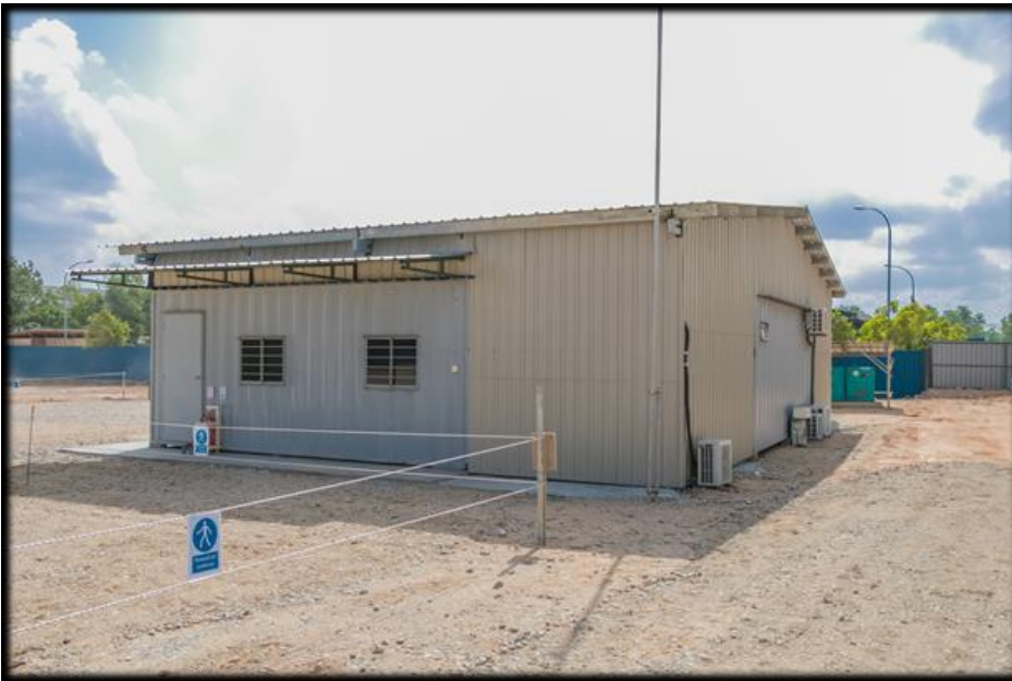
Site construction office
