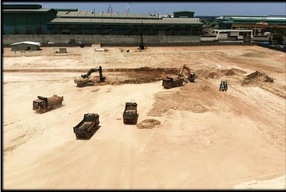
Bulk earthworks and soil removal
