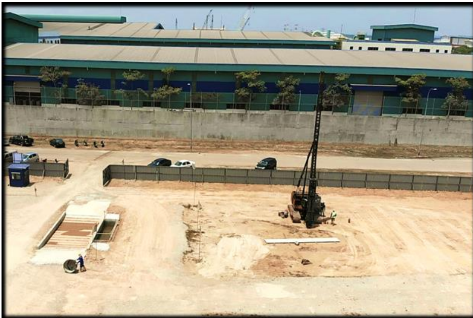
Foundation piling rig on site for tests
